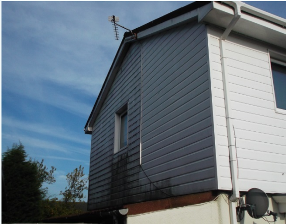
Cleaning of UPVC cladding Glazebrook Rd
